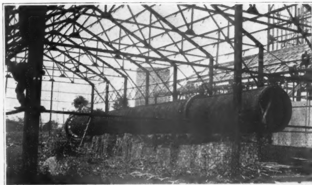
Rotary Kiln in Lime Plant
